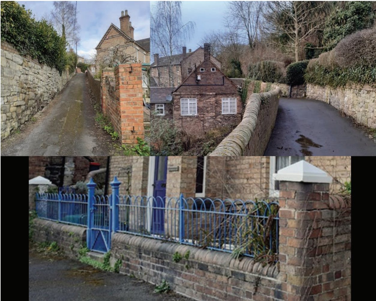
Figure 27: Traditional boundary treatments in stone and brick, sometimes with iron rails and gates, are key characteristics in the street scene
