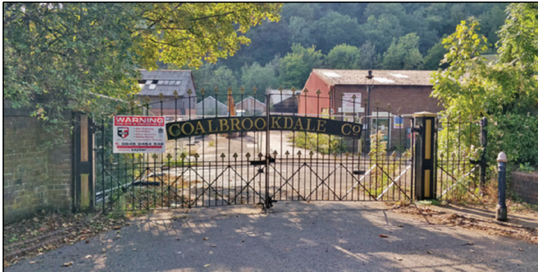
Figure 16: Former Coalbrookdale Foundry
