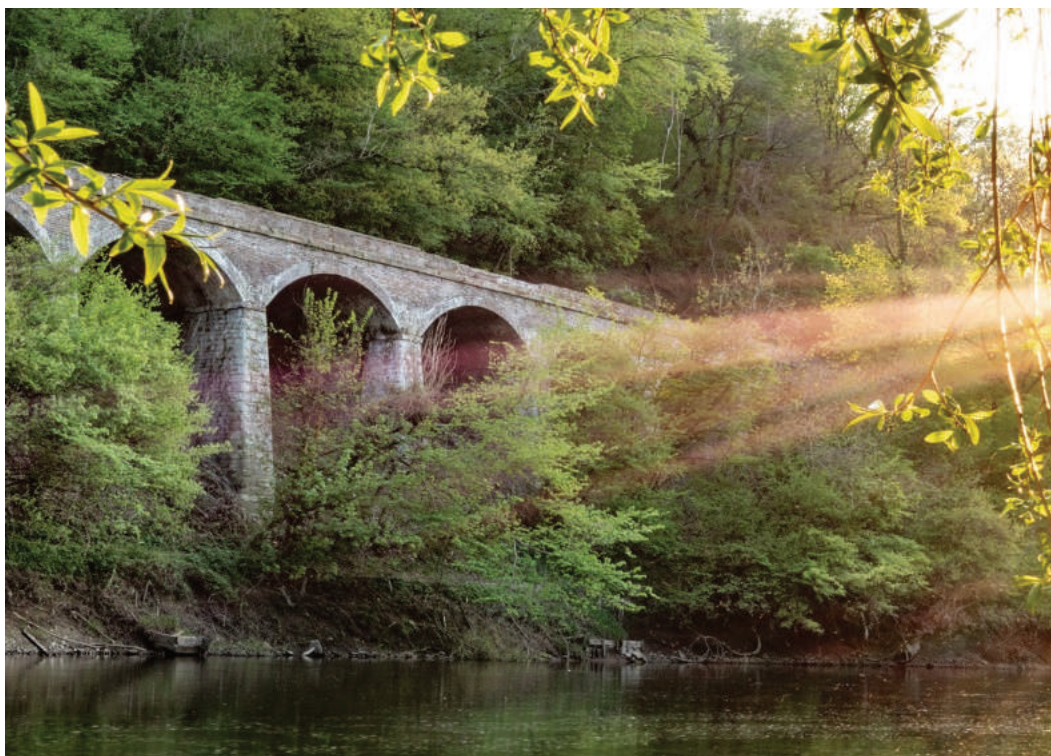
Figure 13: Viaduct at Coalbrookdale
